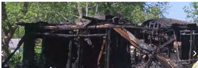
One person died and one was injured in a house fire and possible explosion in Zeigler, Illinois. (Credit: KFVS) https://www.kfvs12.com/2026/04/16/deadly-house-fire-possible-explosion-under-investigation-zeigler-ill/
